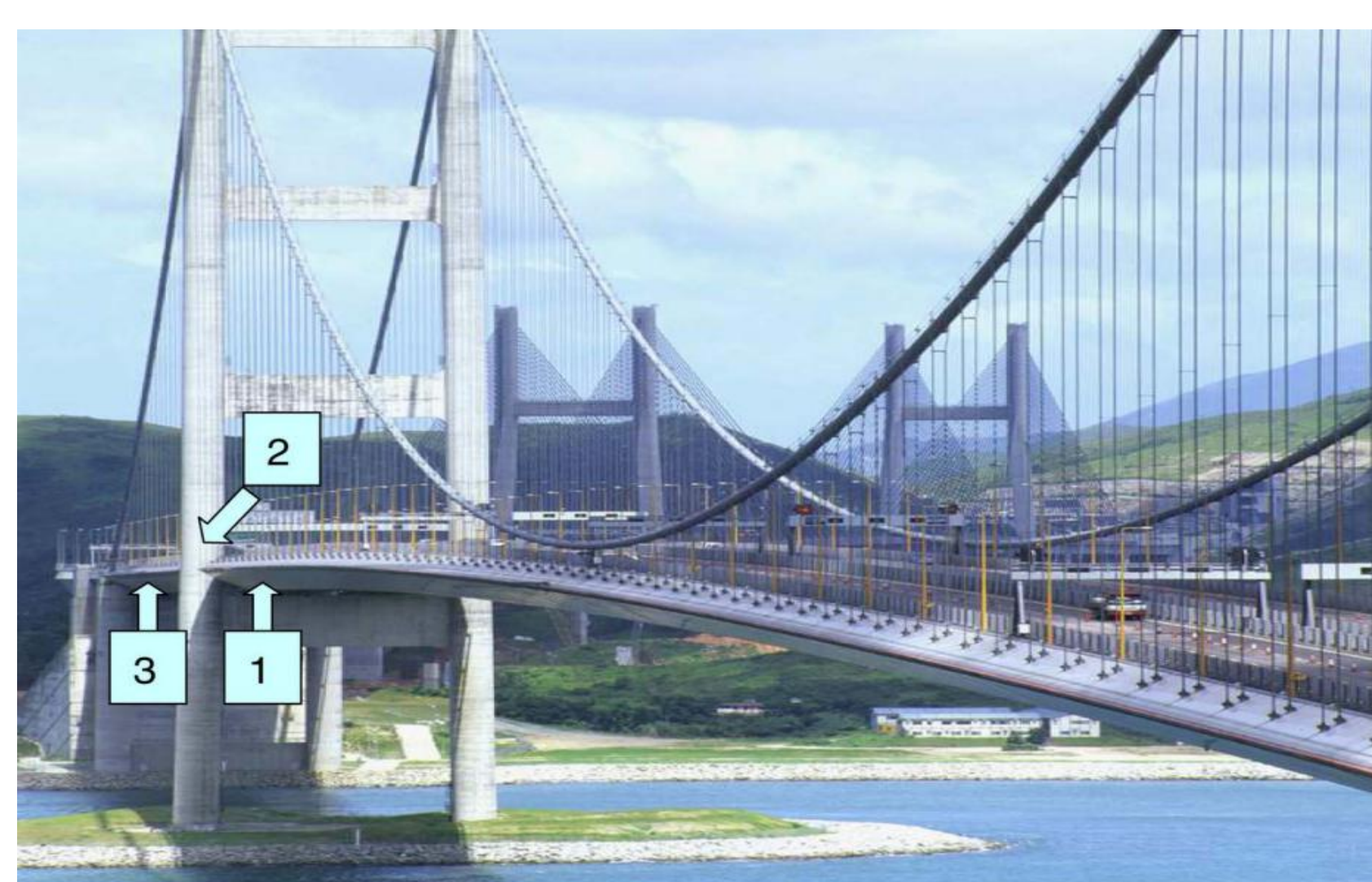
Figure 2. Tsing Ma bridge [4]
